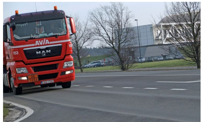
Heavily rutted asphalt pavement, due to heavy traffic and accelerated by high ambient temperatures © FEBELCEM
